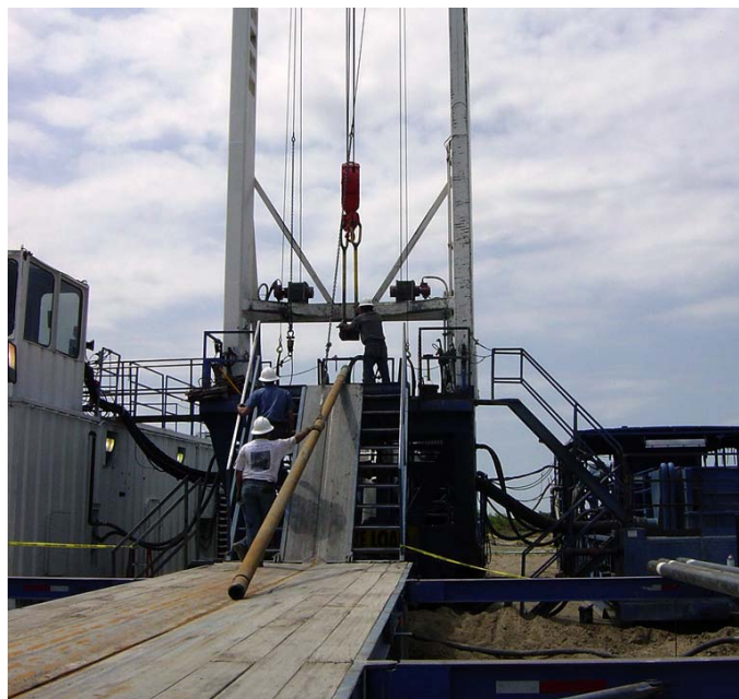
Figure 5: Injector Wheel laid down for BHA & jointed pipe handling.
